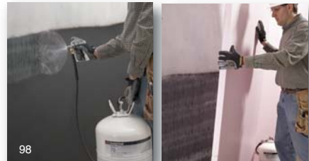
For fast, easy foam board installation above and below grade, simply spray and stick with 3M™ Scotch-Weld™ HoldFast 70 Cylinder Spray Adhesive. Bonds foam to concrete, waterproofing, OSB, and more without damaging the foam.
