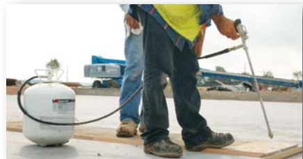
3M™ Scotch-Weld™ Cylinder Spray Adhesives help improve speed and productivity for tilt-up contractors. Just spray and adhere reveal strips, shoe plates, chamfers and inlays to the casting slab without nailing or mechanical fasteners.
